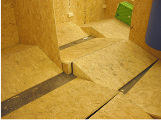
(a) floor with slope.
